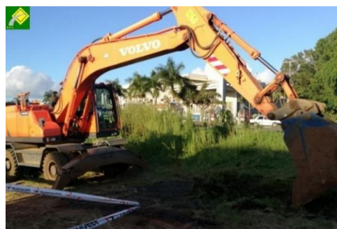
Construction of A1-A3 link Road
