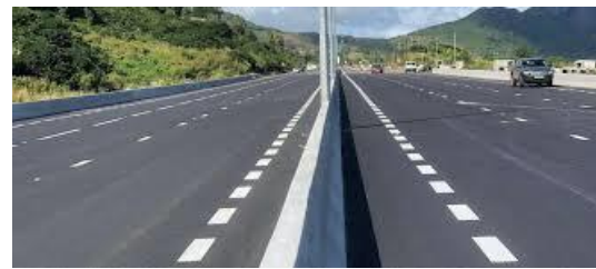
Repairs to embankment failure Terre Rouge Verdun
