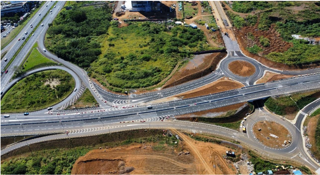
Interchange construction and Improvement along M3-A14 corridor at Ebene
