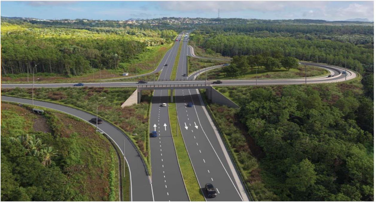
Construction of a Flyover on Motorway M1 at La Viege
