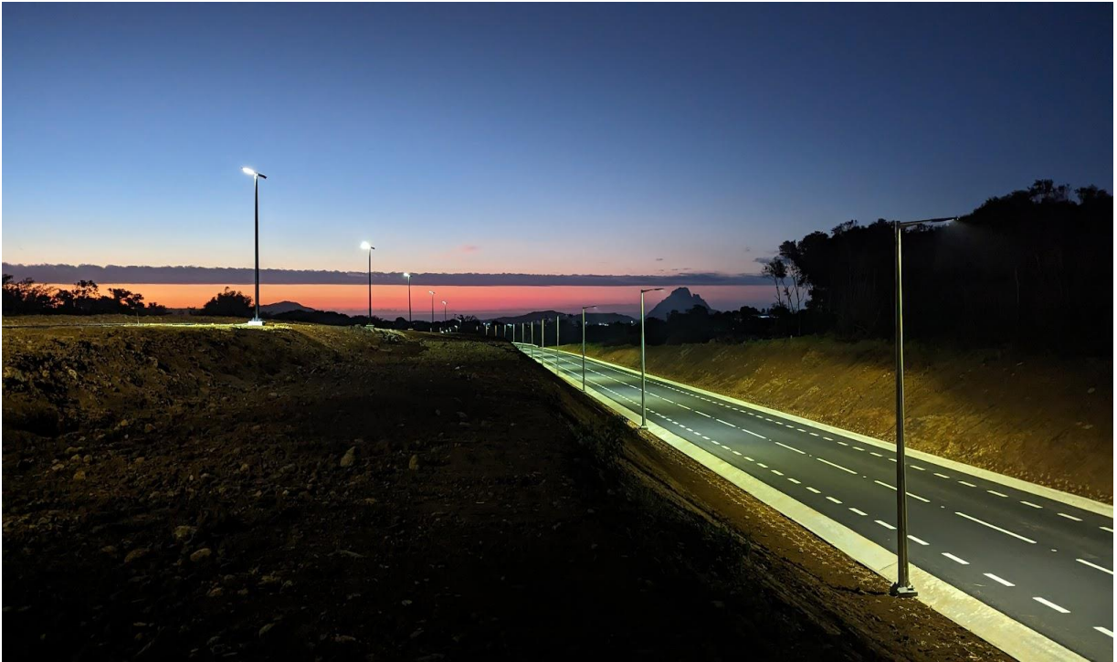
Construction of La Vigie La Brasserie Beaux Songes Link Road - Phase 1
