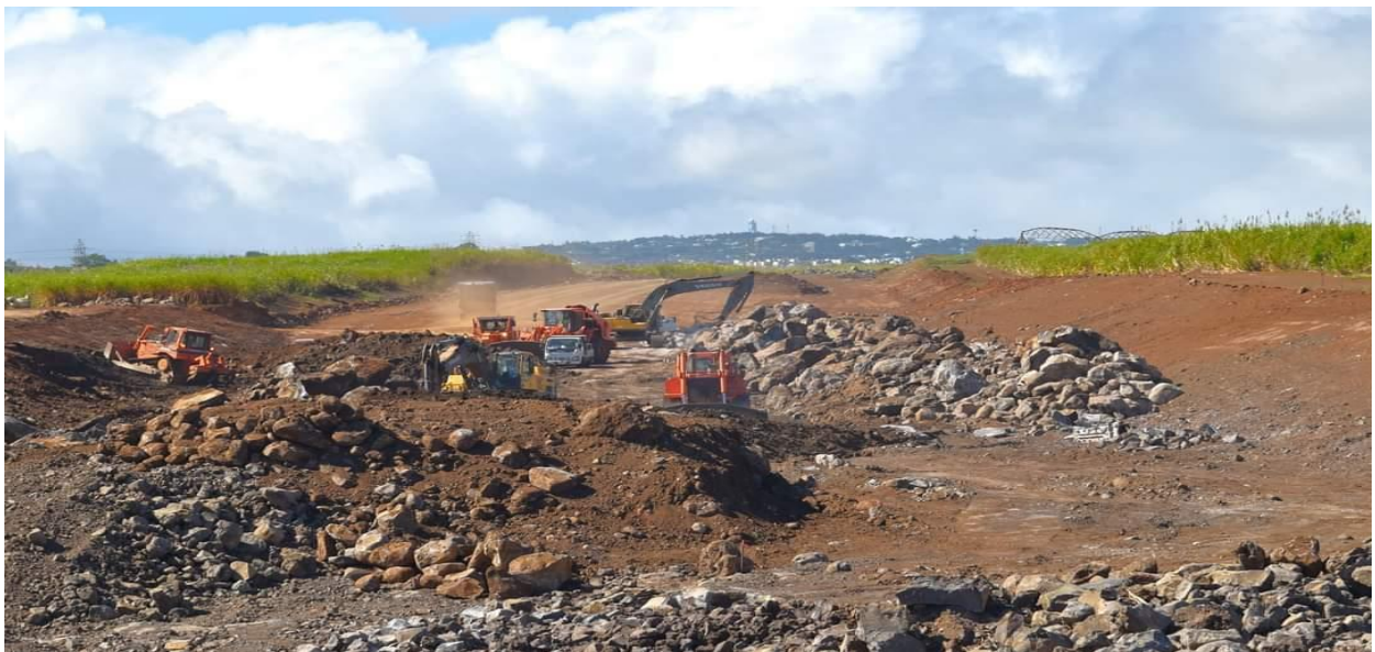
Construction of Flic-en-Flac bypass from Xavier to Pierrefonds
