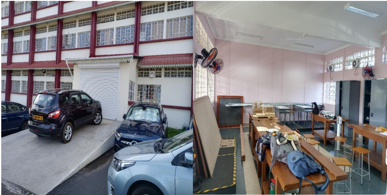
Conversion of existing classrooms into DC/DT workshop with furniture and drawing room
