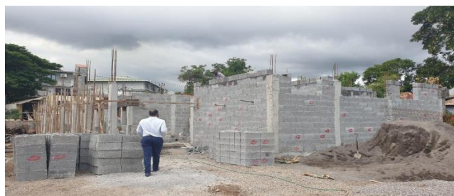
Construction work of a Sub office at Cassis Furniture
