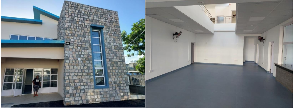
Construction of full-fledged CHC with amenities with parking and fence
