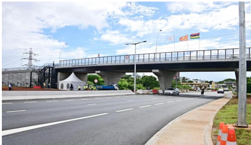
Quay D Flyover
